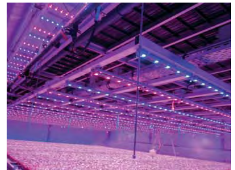
Figure 7. Plant growth unit employing LED grow lights. Photo: PlantLab R&D, NL.
