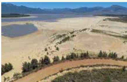
➤ Theewaterskloof Dam in the Western Cape is a major supplier of water to the Cape Town metropole and surrounding areas which include vast tracts of cultivated lands. Decreasing rainfall in the catchment area has resulted in serious consequences for water usage by consumers including agriculture. Source: www.ewn.co.za.
