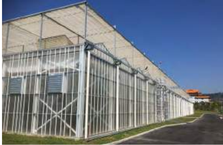
› CH Biotech Greenhouse Facility equipped with an advanced Smart Control System.
