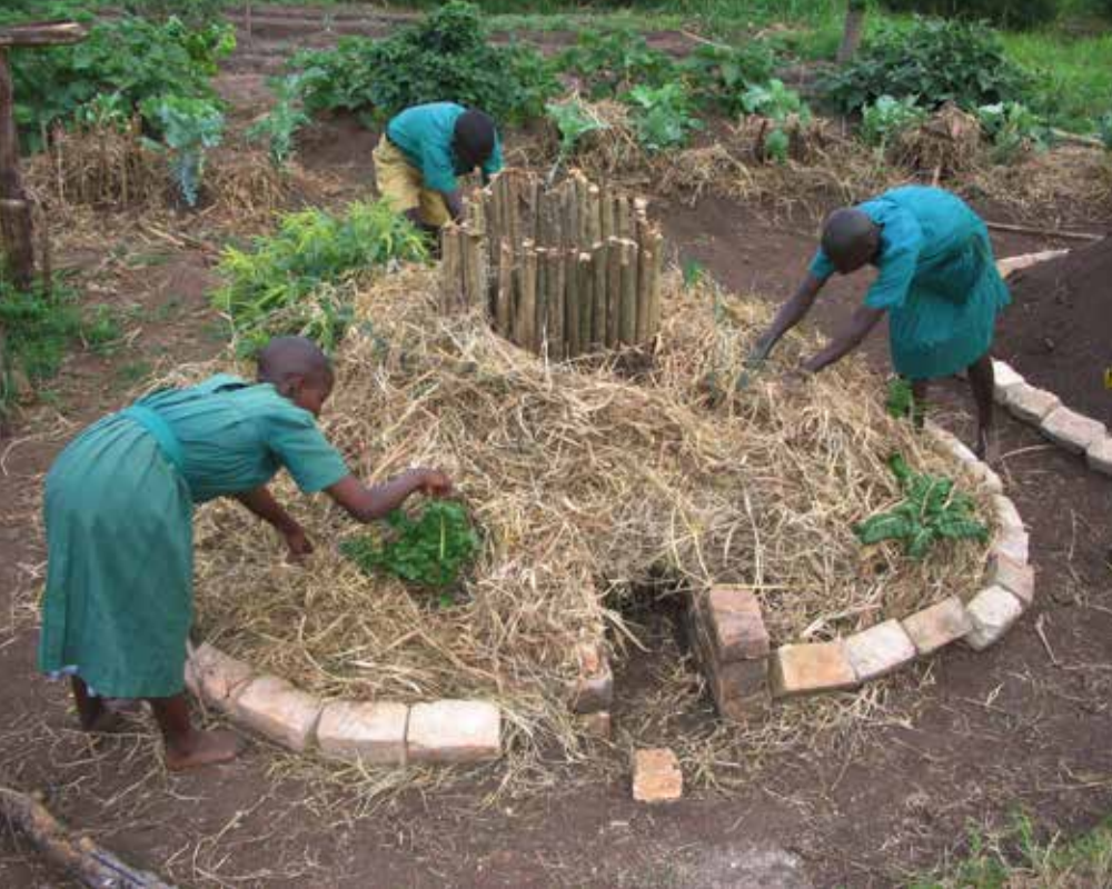
■ Figure 2. A keyhole garden is a circular structure with raised sides often used in Africa for growing vegetables. Photo from: Send a Cow, www.sendacow.org .
